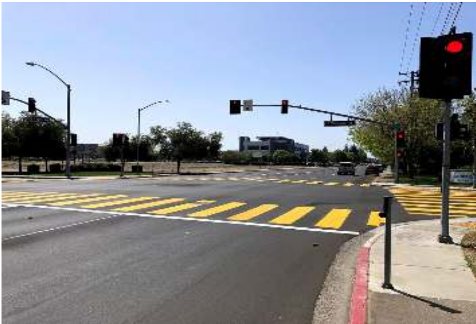
Pavement treatment and new striping at Olive Ave./Tuolumne Rd.
