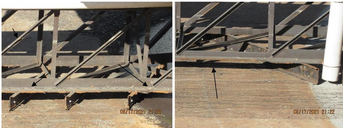
The rake arms are exhibiting edge corrosion on about 10% of the structural steel. This is active isolated corrosion that will cause metal loss. The scraper blades on the bottom has active corrosion.
