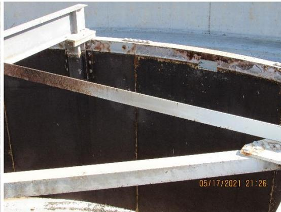
The feed well and supporting structural steel is exhibiting isolated corrosion that can lead to pitting due to metal loss.
