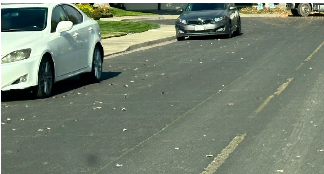
Photo 1: Section 1 Moderate Longitudinal Cracking
